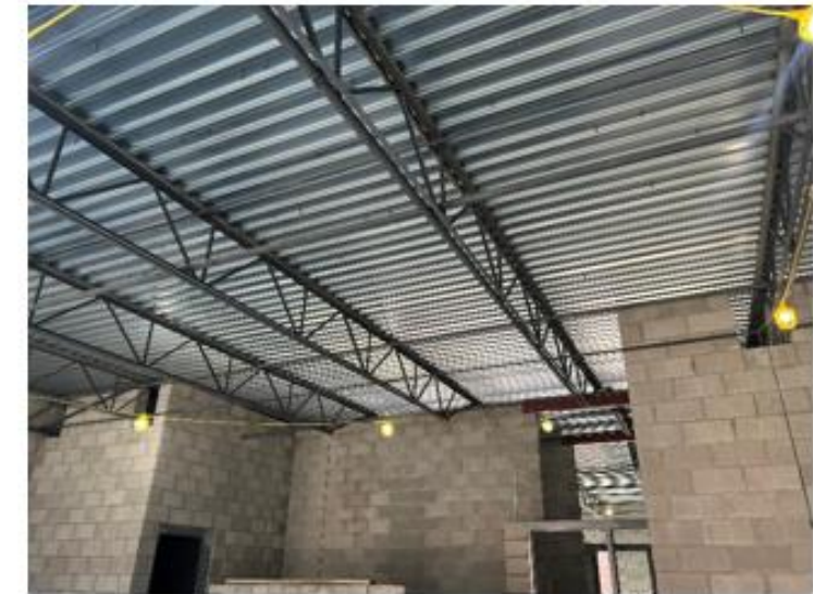
Roof decking over classroom addition
