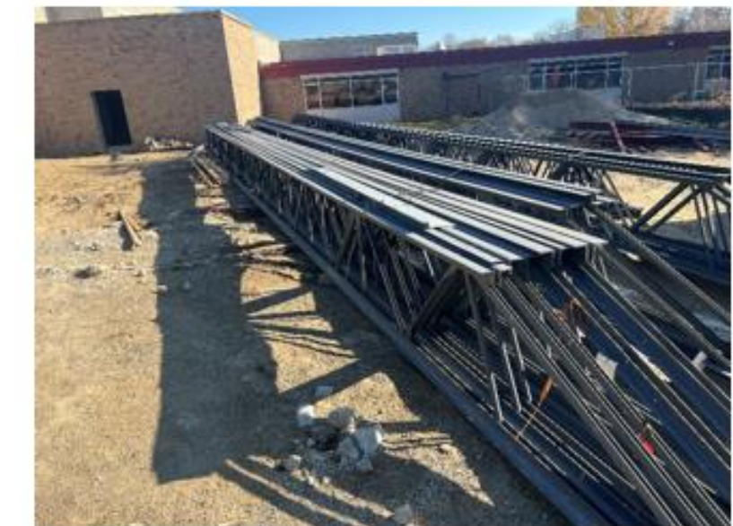
Steel joist ready to be installed
