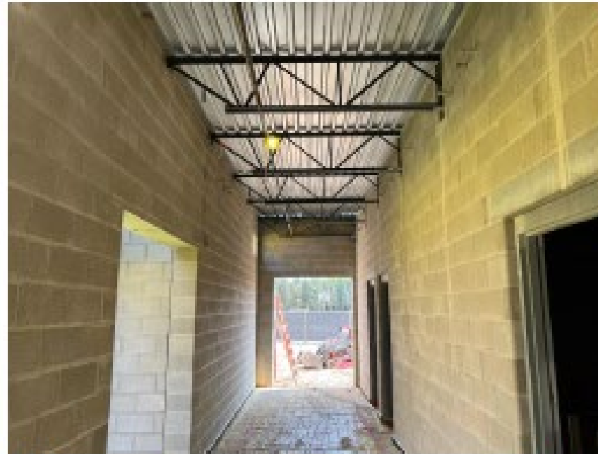
Hallway decking and joists have been installed
