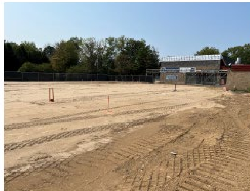
Front addition pad ready for foundations to start
