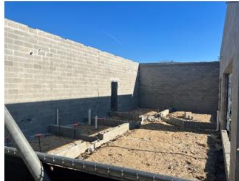
Interior block walls being constructed
