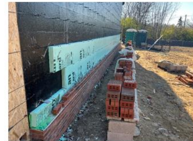
Brick façade being installed
